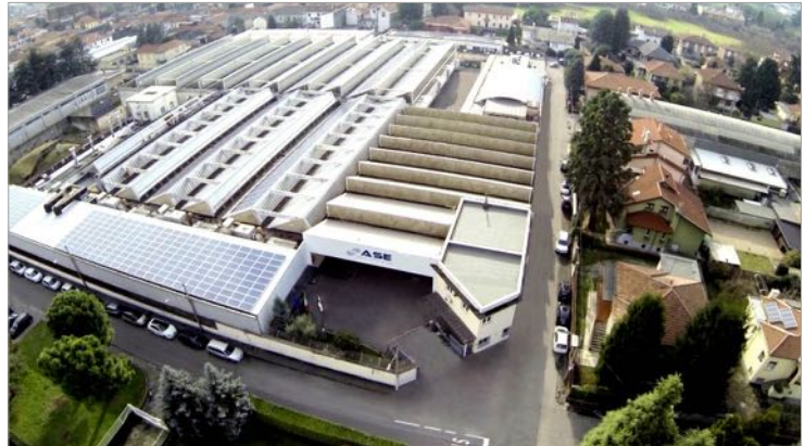
ASE headquarter and operational plant: Aerospace District in Lombardy, near Milan and Malpensa Airport.
